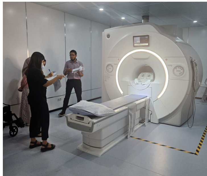
Figure 8. Installation of MRI 1.5 T at Bahtera Mas Hospital
