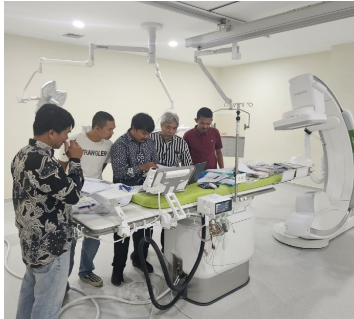
Figure 7. Installation of Cathlab
