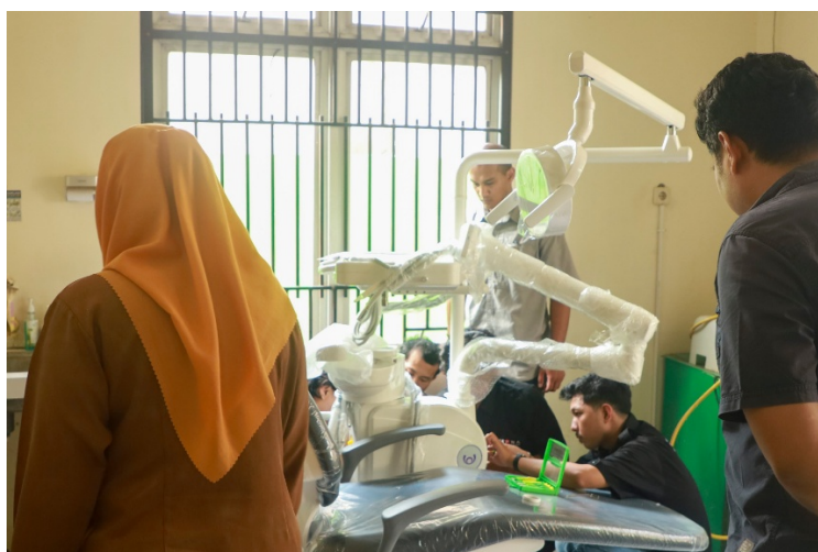
Figure 6. Installation of Dental Chair at Public Health Center
